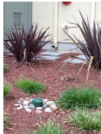
Roof runoff is directed onto landscaping for infiltration in San Jose
