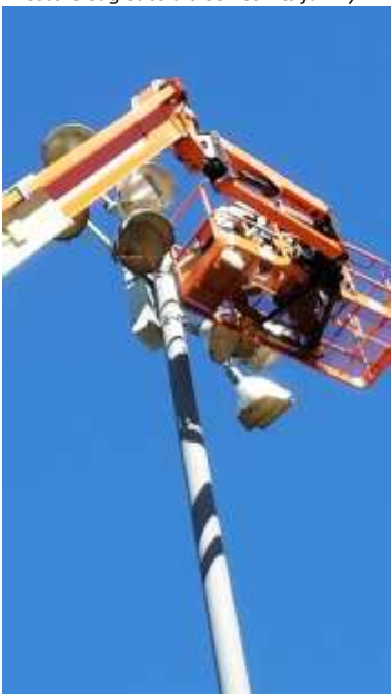
Public Works staff replace field lights at the Milpitas Sports Center
